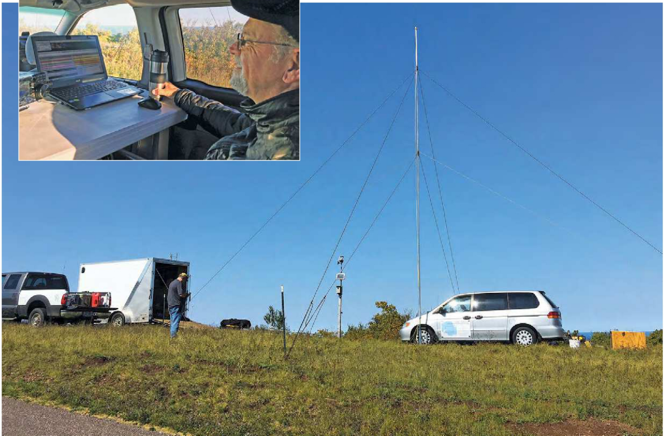
Erection of the 35-foot mast with drive-on plate and multiple guy ropes. On the side of the van is the banner created per the sign posting agreement, declaring the team's amateur radio activation of EN67 and the hours of operation.
